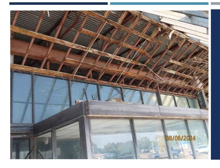
VIEW UNDER THE AWNING SHOWING COLLAPSING BOARDS AND RUSTED BEAMS.
